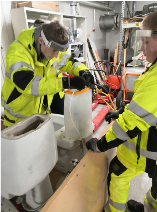
In the picture, the students are practicing the maintenance of the toilet seat.
